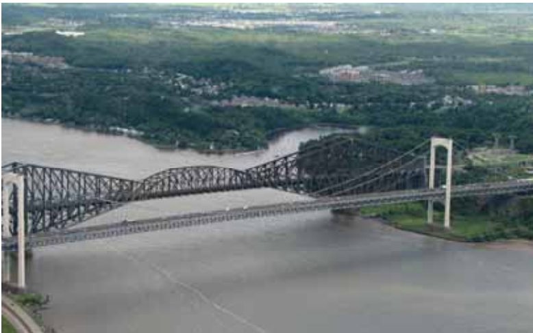
Pont de Québec is the longest cantilever bridge span in the world.
